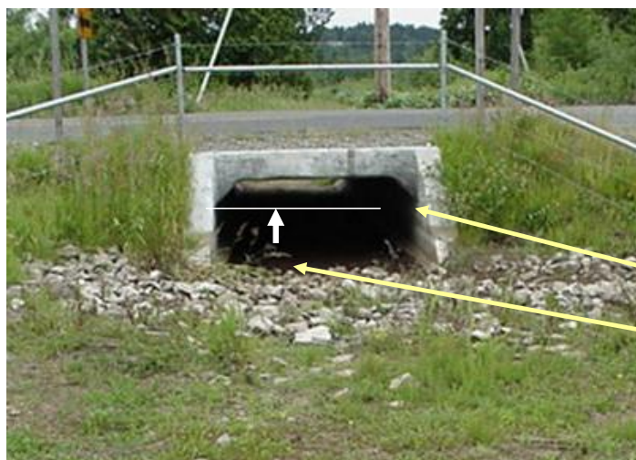
Figure 22: A box culvert that is the outlet of a depressional wetland. The live-storage is measured as the distance between the bottom of the culvert and the water marks on the side. The distance is approximately 15 inches.
